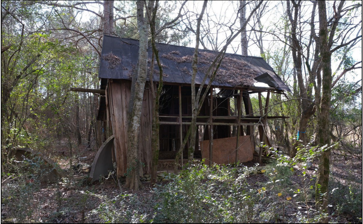
Figure 16. Southerly View of Structure at 9BR1289.
