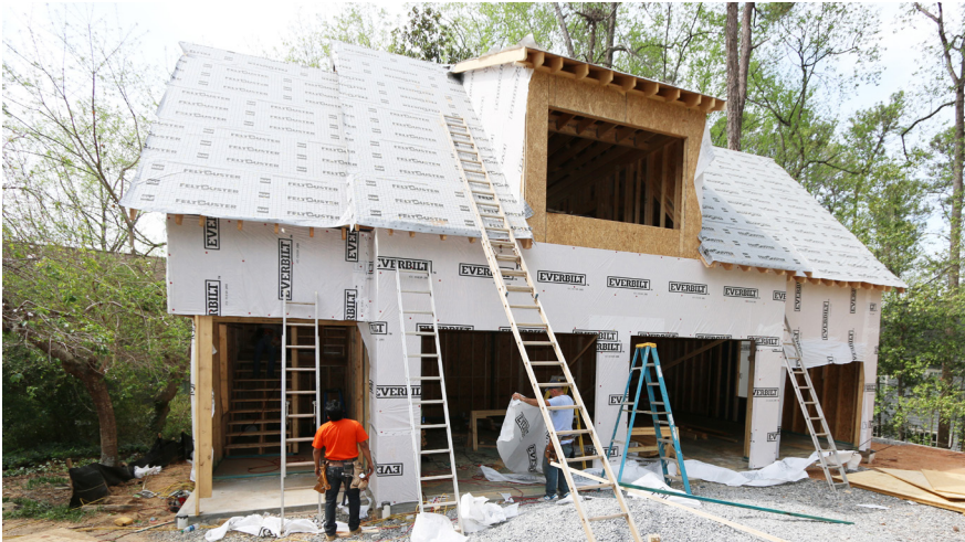
352 HERRINGTON DRIVE NEW CONSTRUCTION
