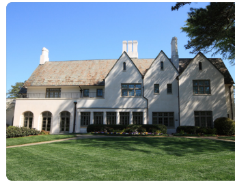
Cherokee Town Club - Renovation Atlanta, Georgia Cherokee Town & Country Club
