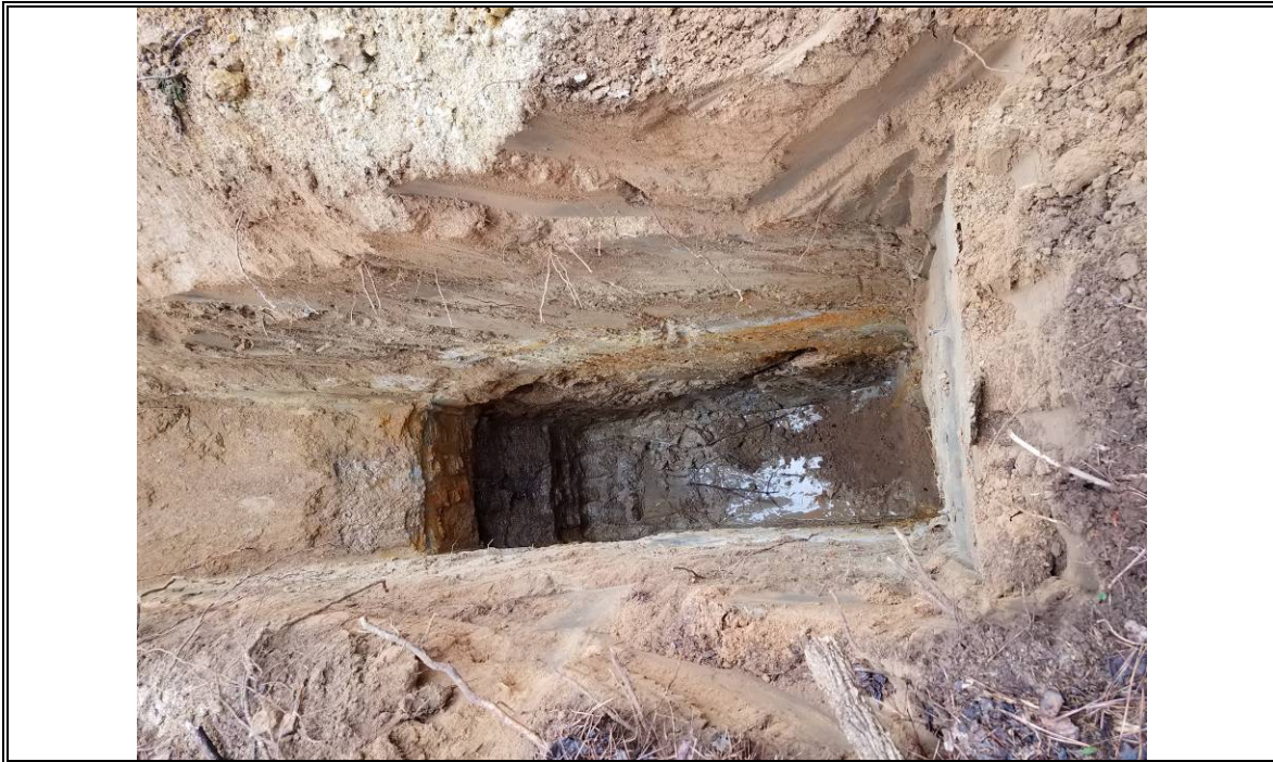
Photo # 5: Test Pit TP-3
