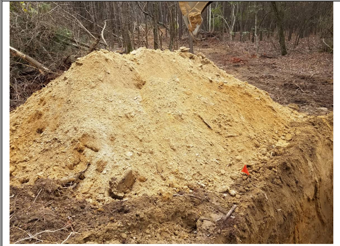
Photo # 2: Excavated Soil from TP-1
