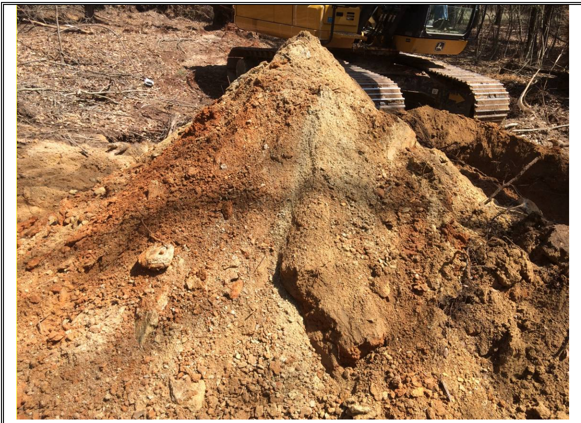
Photo # 28: Excavated Soil from TP-13A
