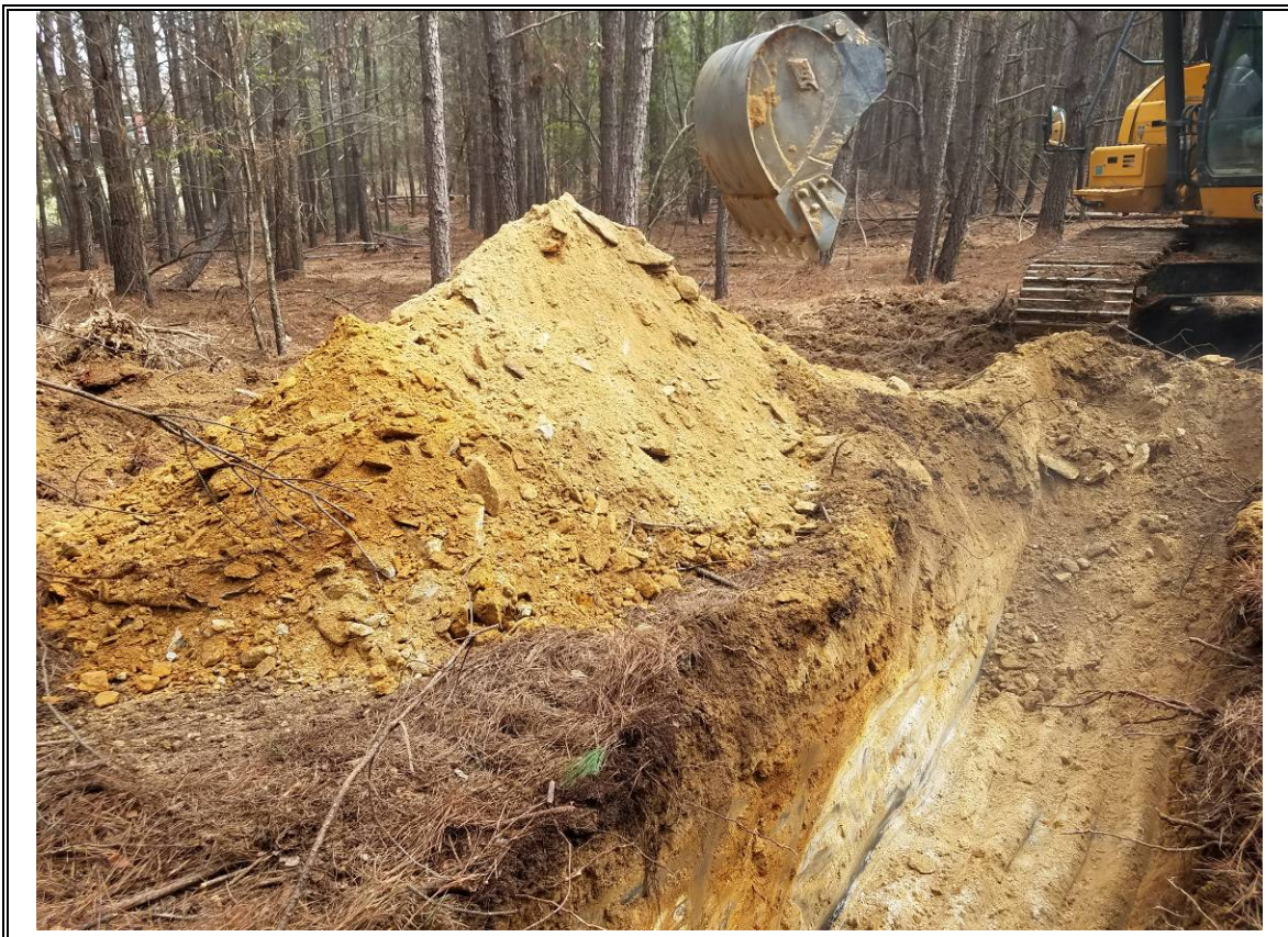
Photo # 14: Excavated soil from TP-7
