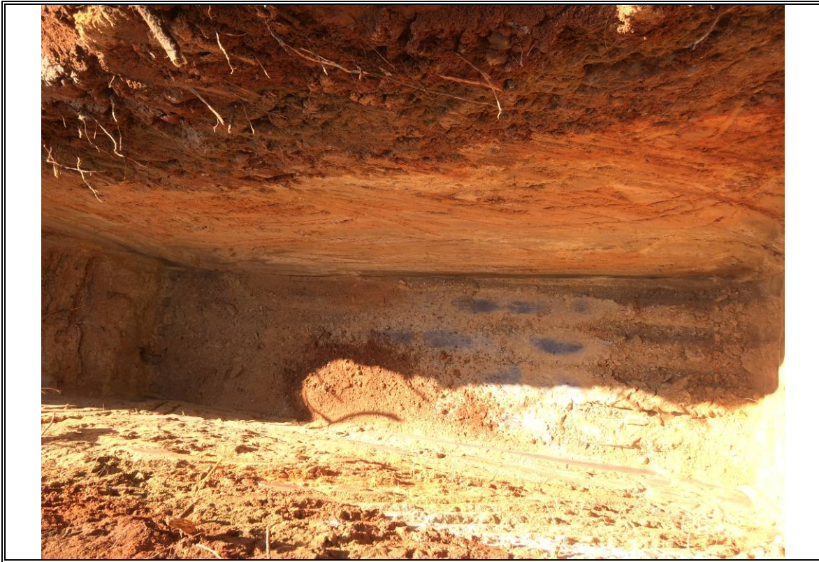
Photo # 15: Test Pit TP-8
