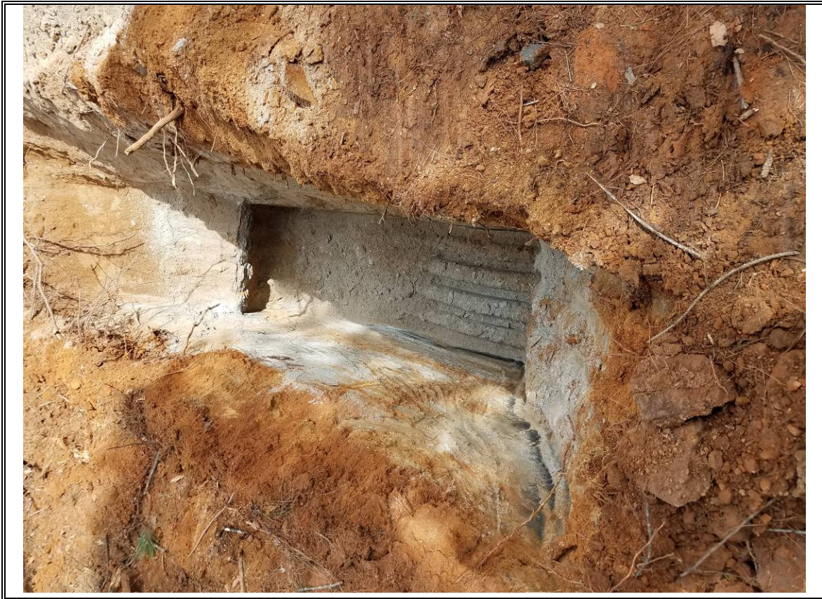
Photo # 21: Test Pit TP-11
