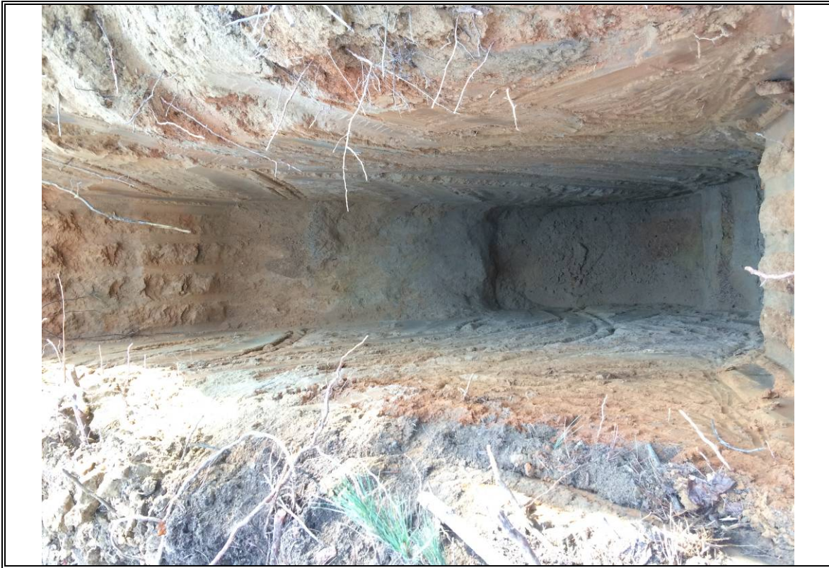
Photo # 43: Test Pit TP-20
