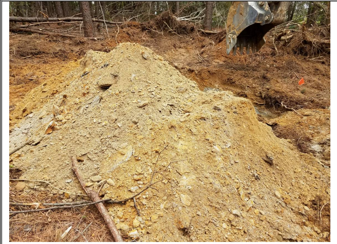
Photo # 10: Excavated soil from TP-5
