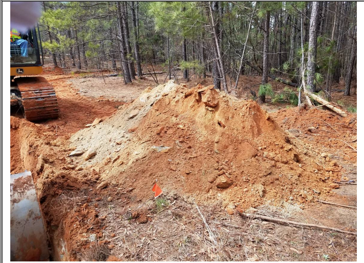
Photo # 24: Excavated soil from TP-12
