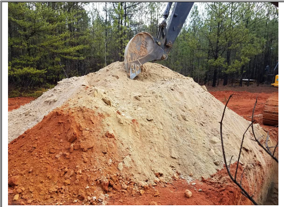
Photo # 32: Excavated Soil from TP-14
