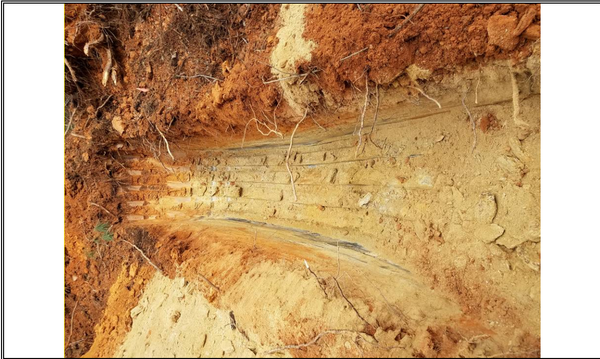
Photo # 19: Test Pit TP-10
