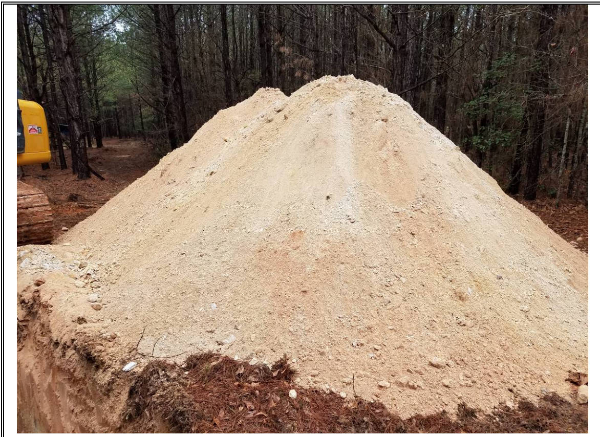
Photo # 18: Excavated soil from TP-9
