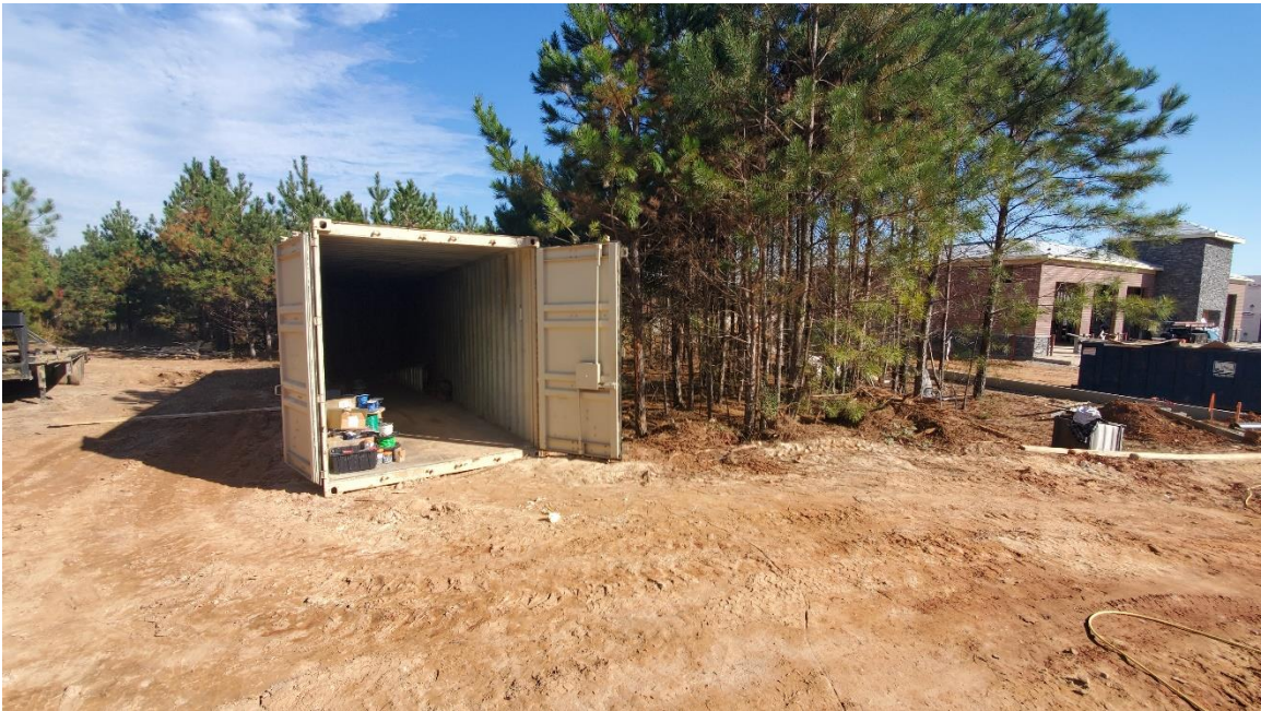
Figure 6- Storage for materials and equipment.
