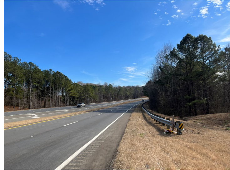
Photo 2: View South along Hwy 515 from Northeastern property boundary
