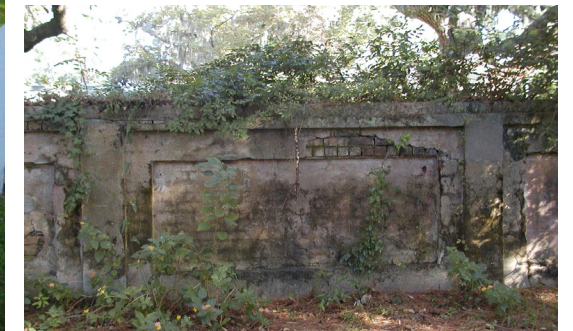
Aged brick wall
