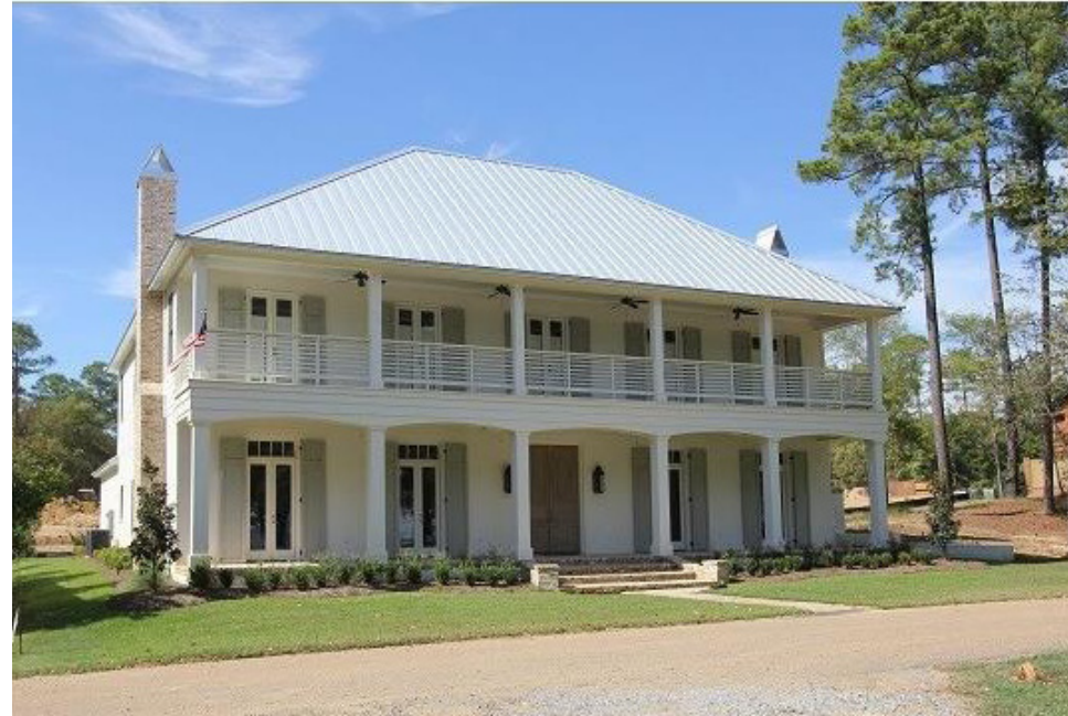
Roof proportion used to express style.
