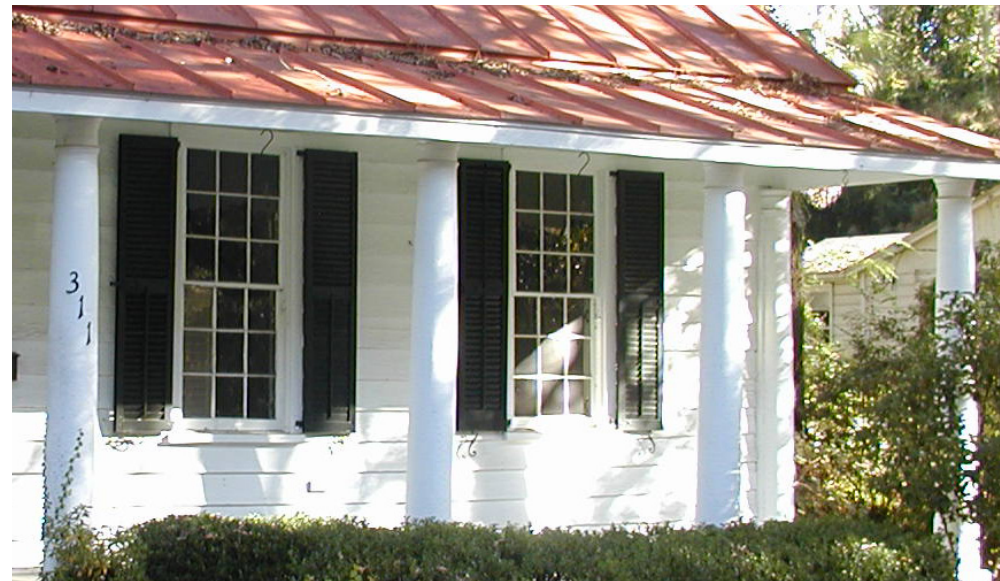
Shutters are being held back with shutter dogs
