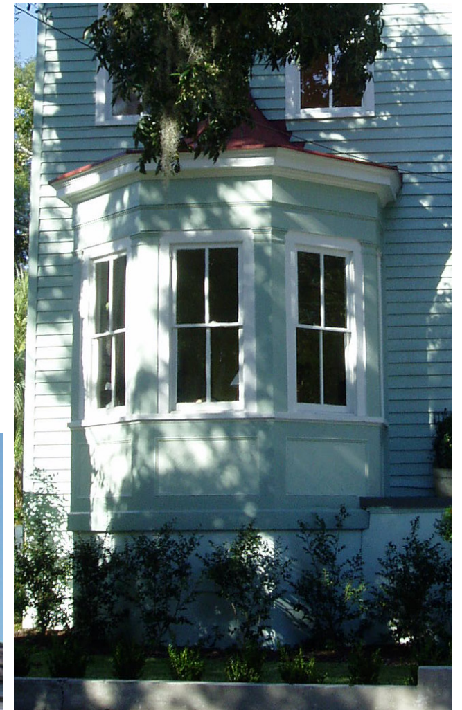
Bay window with proper execution
