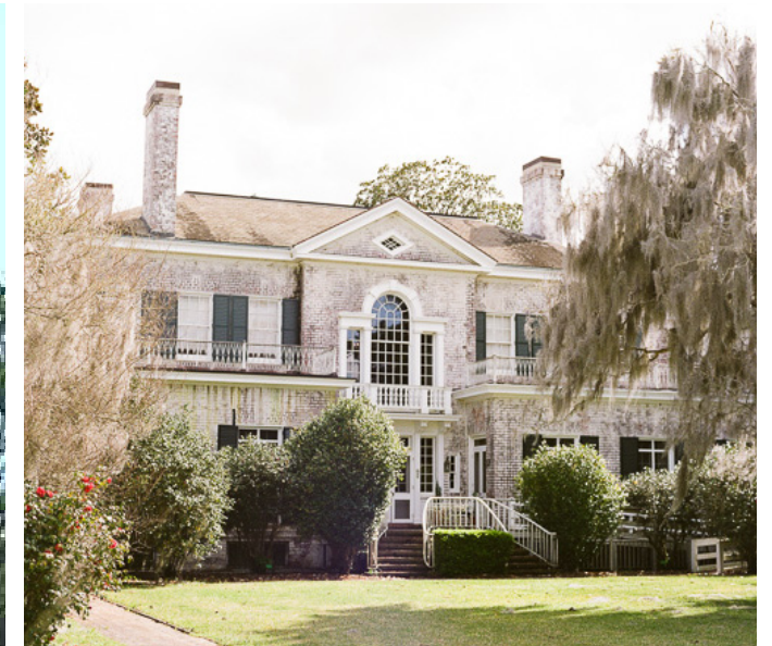
Brick Foundation and Chimneys
