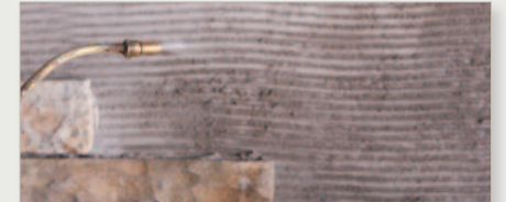
Moisten the scratch coat and the back of the Stone, especially in hot or windy climates
