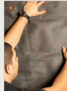
1 Install Water Resistant Barriers. (exterior applications)
