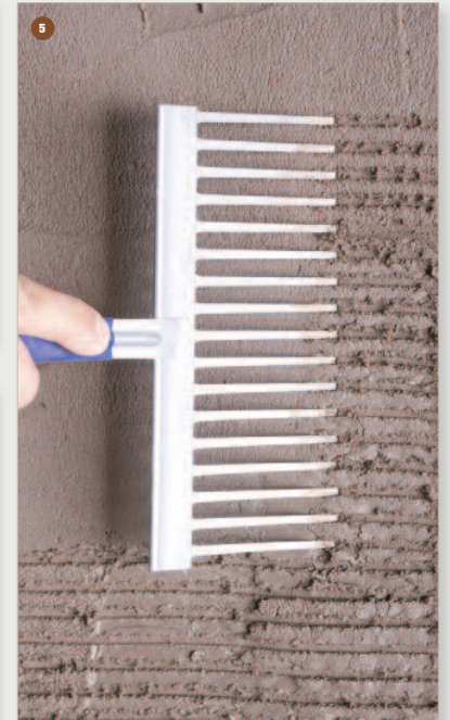
5 Rake mortar to create scratch coat.
