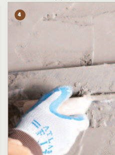
4 Apply mortar for scratch coat.
