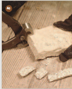
4c Trim stones to fit. Option C - Nippers
