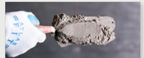
Mortar Consistency is best for application when it starts to stick to your trowel.
