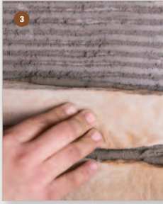
3 Install flat stones.
