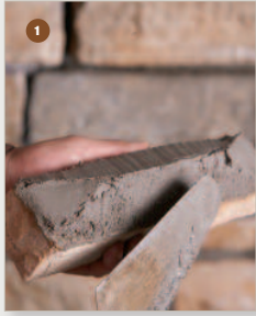
1 Apply mortar to the entire back of the stone.
